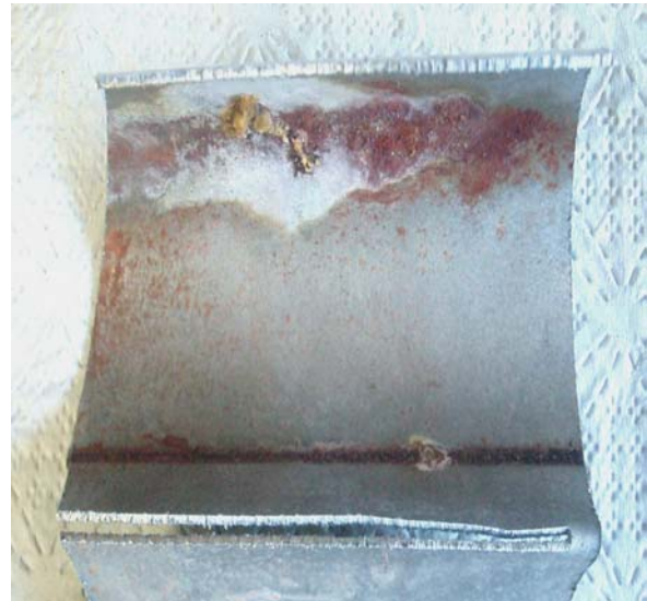
Figure 3: Oxidized Aluminized Steel Tube I.D. Section
